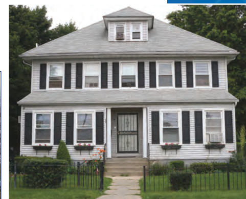
Edna Moran INN, Emergency Family Shelter
