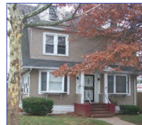
Donald Axinn INN, Emergency Men's Shelter
